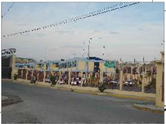
3 TERMINAL TERRESTRE COLLASUYO
