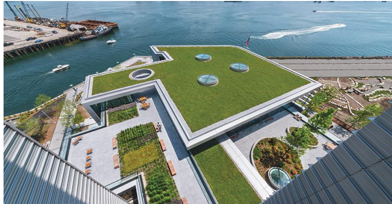
Figura 75: Vista de Techos verdes Spaulding Rehabilitation Hospital
