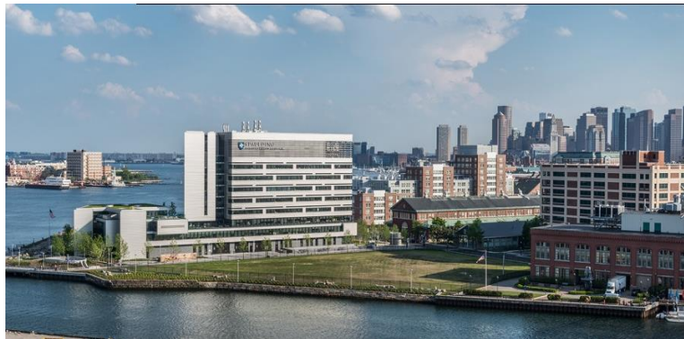
Figura 66: Spaulding Rehabilitation Hospital: Bahía de Boston, Massachusetts
