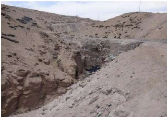
Riverbed of the Devil’s Creek obstructed by an informal em- The place of the informal embankment collapsed by the bankment as an access trail to farms on the Alto de la Alianza flood of 22 February 2020 and that caused the flood to- wards the city of Tacna. Source INGEMMET (2016). wards the city of Tacna.
