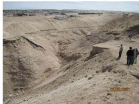
Riverbed of the Devil’s Creek obstructed by an informal em- The place of the informal embankment collapsed by the bankment as an access trail to farms on the Alto de la Alianza flood of 22 February 2020 and that caused the flood to- wards the city of Tacna. Source INGEMMET (2016). wards the city of Tacna.
